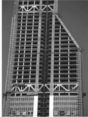
Figure 11.3 Multiple antennas in a large building.
