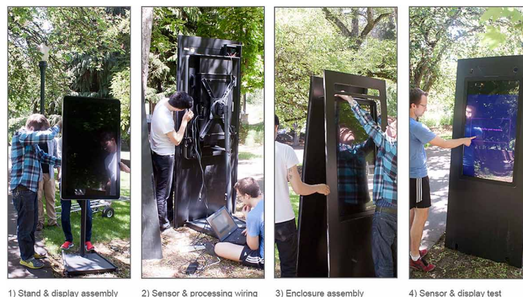
Figure 7. Field assembly and final test bed
