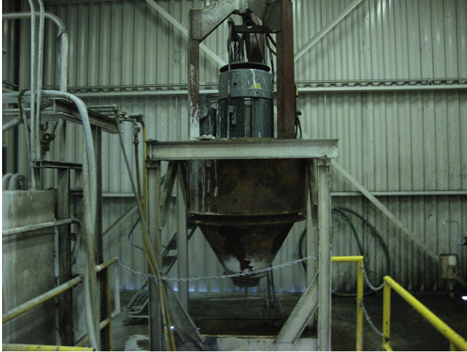
Figure 8.4 Dry scrubber atomizers.
